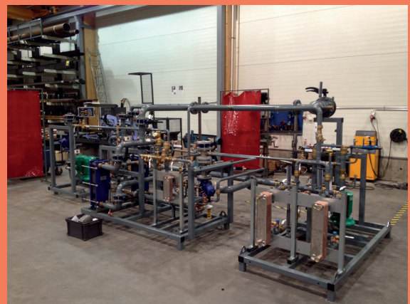
2 out of the 9 heating substations before delivery to Expoforum
